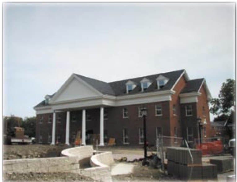
The Texas Delta Chapter House Nearing Completion 10/13/05
